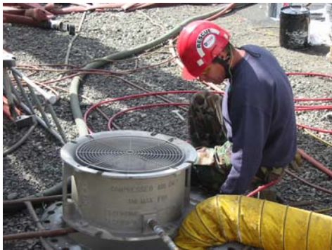
Perennial Power: Confined Space Rescue Standby June, 2006 and June, 2007
